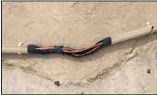
Figure 3.9: The DC power cables are lying on the roof/ground exposed to external interventions.
