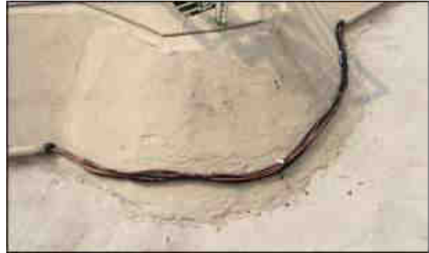
Figure 3.9: The DC power cables are lying on the roof/ground exposed to external interventions.
